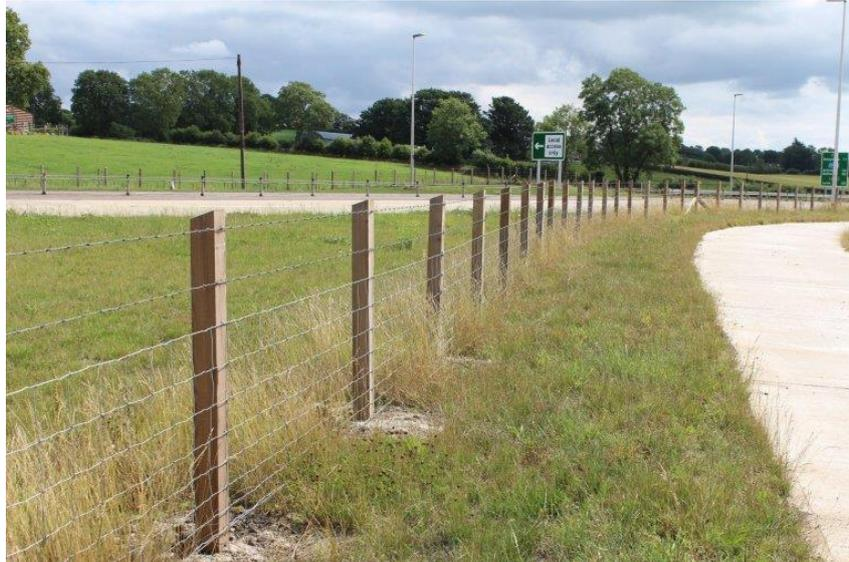
Figure 6: Timber post and wire fence
