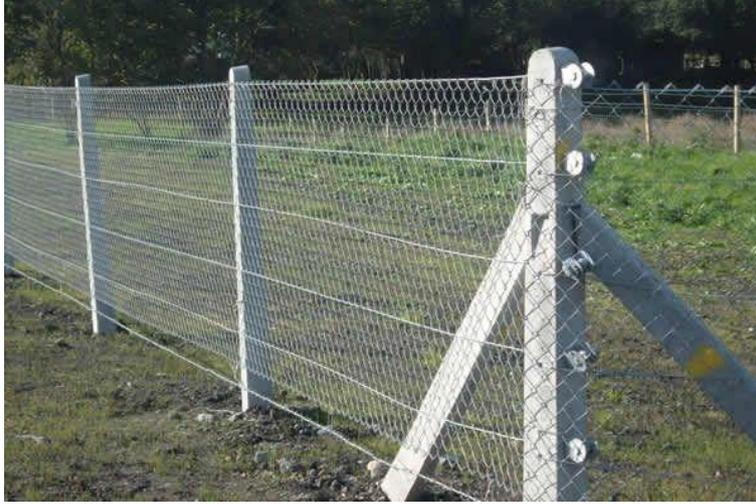
Figure 5: Concrete post and wire fence
