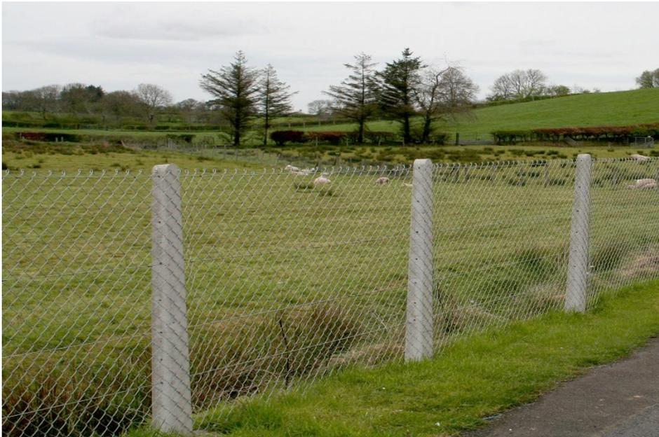
**Figure 4: Concrete post and chainlink fence**
